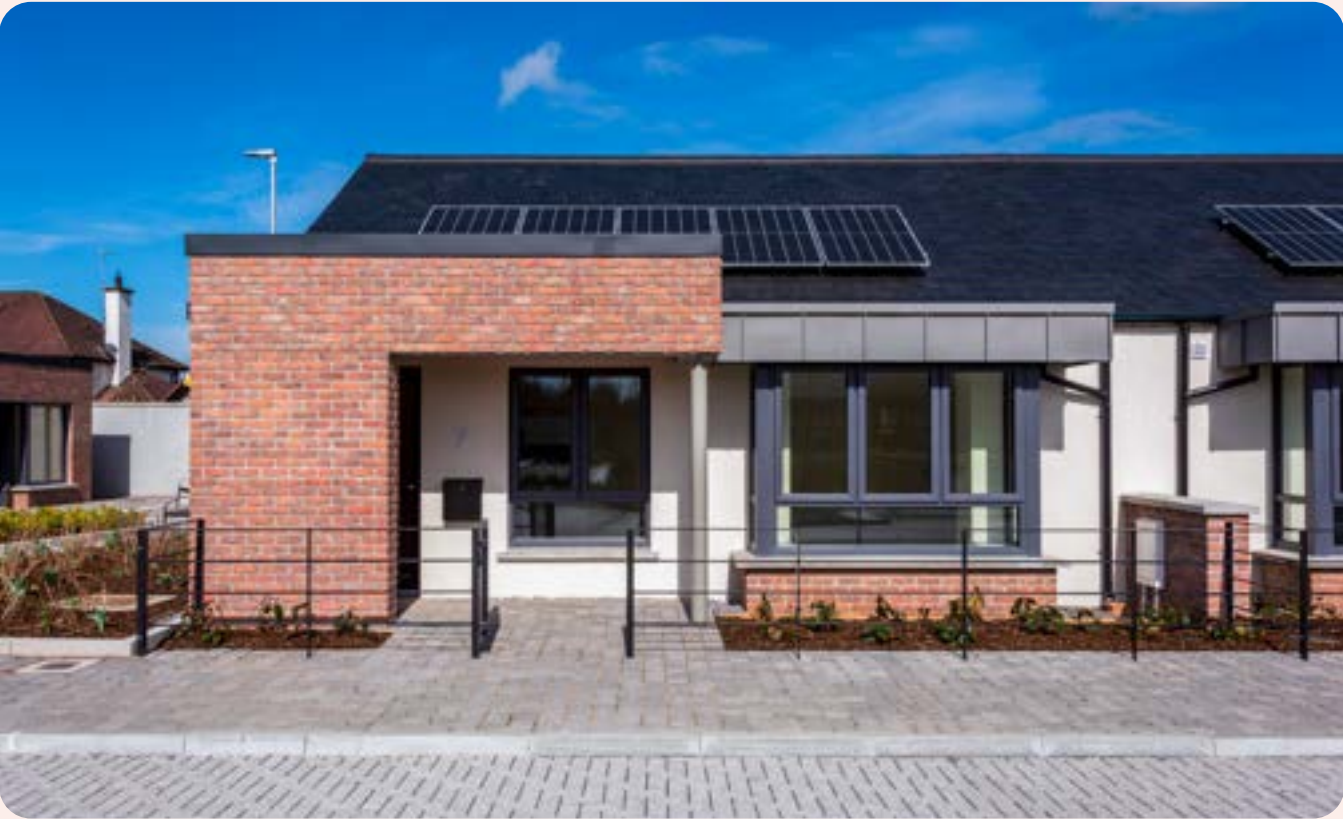
Clonminch, Social Housing Development Award Nomination
